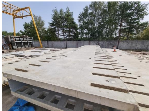
Production of LCCs at Mace's offsite factory in Brandon
