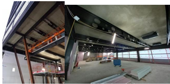
Fully installed LCC in Block A (Office) Palmerston Court
